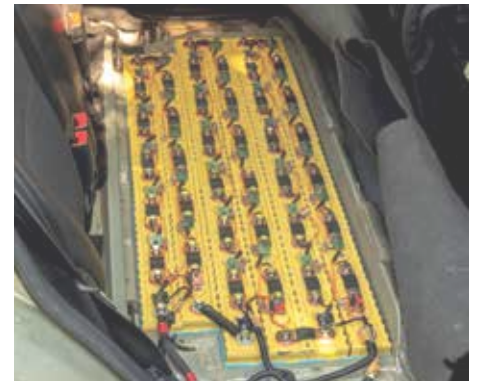
Large and/or unattended battery storage areas
