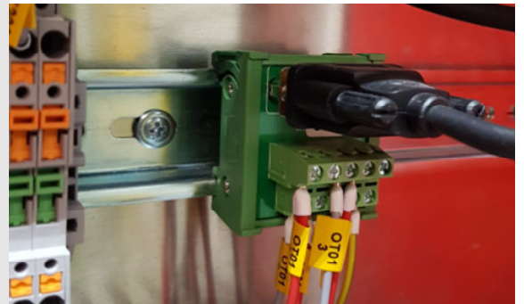
DB9-Screw Terminal adaptor for DIN Rail Mount
